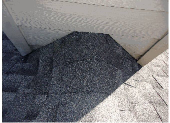
Exterior: View behind chimney - OK
