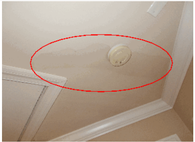
Stain near attic pull down - no moisture detected
