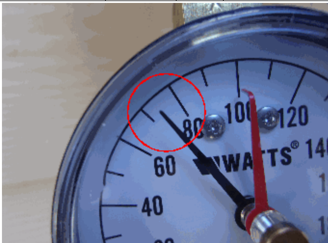
Water pressure at outside spigot
