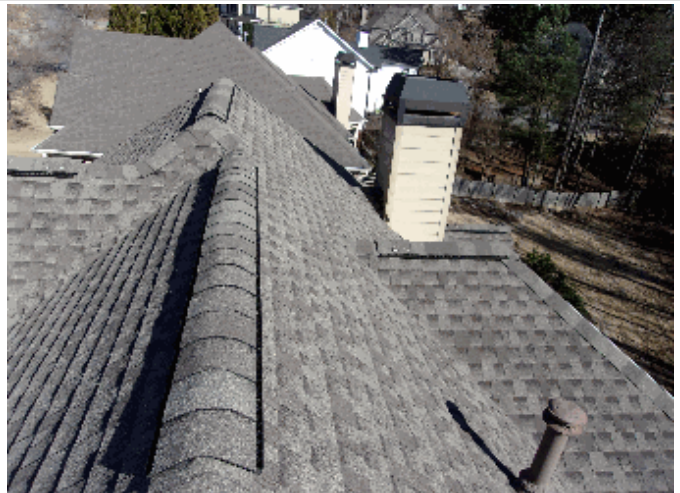
Overall view of the roof
