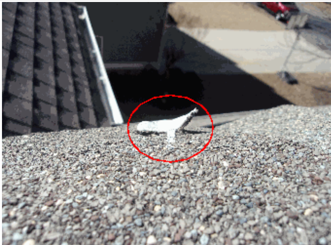
Areas of the roof will need to be resealed periodically
